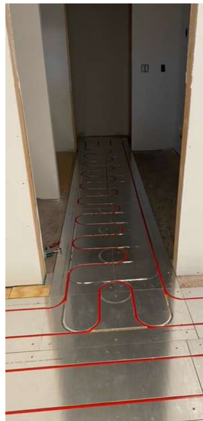
Above: Note the creative tubing layout designed to route tubing from the room down this narrow hallway.
